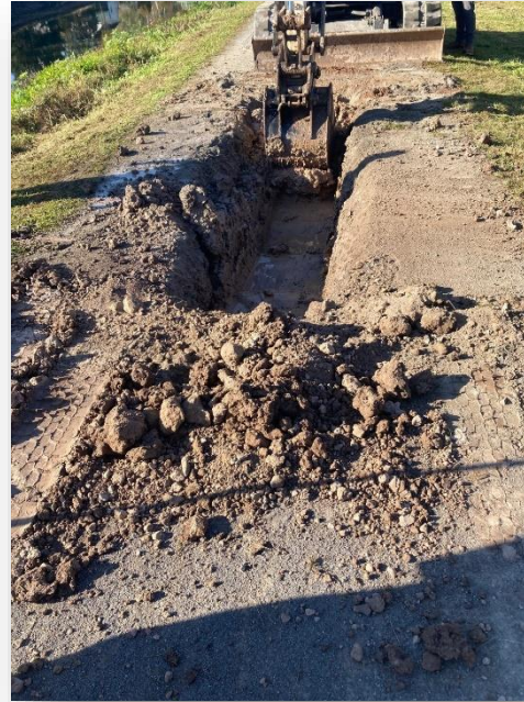
Clay Cut-Off Wall Installation
